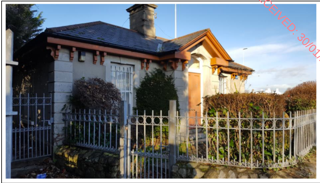
Figure 2.3 - Front of the Gate Lodge
